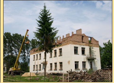
Raising the roof
